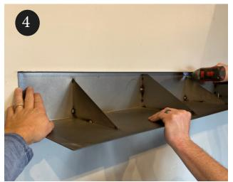
Using two people hold base up to line and pre-drill holes with a small drill bit ( not included) and then use screws (provided) to mount base to wall. Be careful to assure you are screwing into the center or studs of other solid backing system. Base should be tight to wall.
