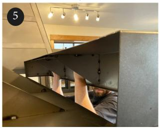
Using two people slowly and gently slide the mantel cap in place onto the base. Mantel cap should get a snugger feeling as it gets close to flushing into wall.
