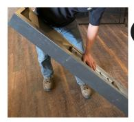
If panels have a bow in them, which can happen in the freight process, they are generally easy to adjust back. Place bowed area across leg as shown and give mild pressure to both sides to conform bowed area back into position. you may have to do this several times with increasing amounts of pressure to get bow out of steel. Do this to both the base and mantel cap.
